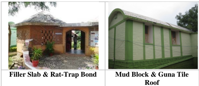
Fig. 2: Rat-Trap Bond with Filler Slab & Mud Block with Guna Tile Roof - Rural Technology Park, NIRD Hyderabad India (Source - Author)
